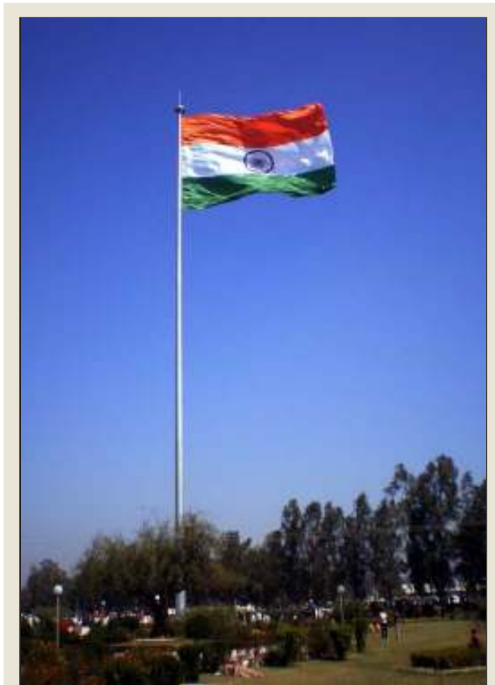
The first tallest flagmast of India with the height of 207ft, weighing 12.5 tons and a 4.5ft diameter at the bottom is at Kaithal, Haryana.
